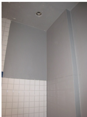
Picture of a bathroom with moisture protection
