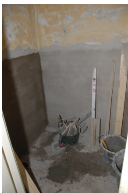
Picture of a bathroom where repair work is started
